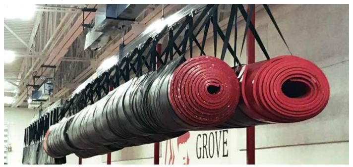
To ensure balanced operation, the Double Mat Lifter unit features a three cable system. Standard lifter, load bar, and slings shall be capable of supporting two standard 42' x 42' (12.8 m x 12.8 m) wrestling mats (weighing approximately 1 lb/ft²). Mats may be one-piece or in sections placed end to end. In case of a power outage, an emergency lowering manual override brake is included. Motors, drive assembly, and all control mechanisms are encased in a fire proof safety cover.
